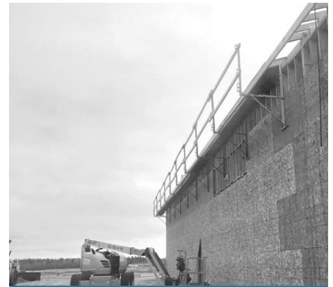
Exterior bracket scaffold being installed
