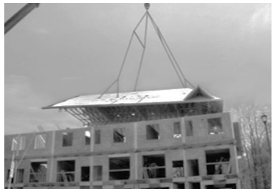
Assembled roof being hoisted into place
