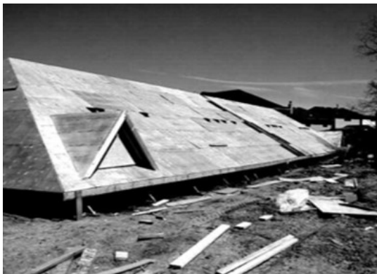
A roof that has been assembled on the ground
