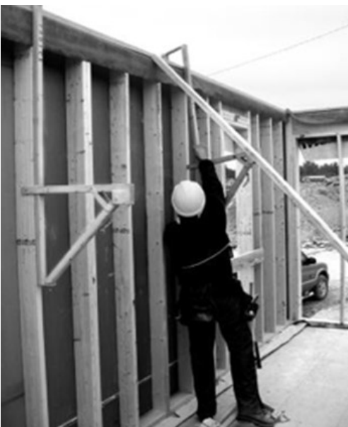
Interior bracket scaffold being installed
