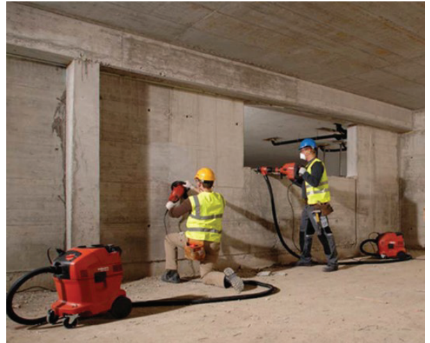
Figure 3 – Using hand tools equipped with dust control solutions
